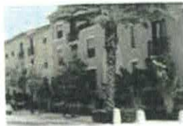
Two to three story Multi-Family buildings with parking garages or structured parking facing an alley
