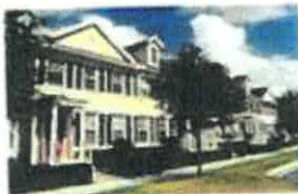
Two story town houses with parking along back alleys
